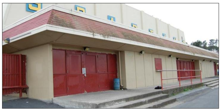
Does this school meet the Good Repair standard? Boarded up windows—but no broken glass (!) ... non-accessible main entrances... moss growing on the roof... downspout dumps on the concrete landing...sloppy paint job, but no graffiti(!)
